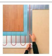
T2Reflecta and T2Red floor heating system consists of an insulated aluminium profile T2Reflecta and the self-regulating T2Red heating
