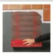
Self adhering, low profile floor heating mat for installation immediately under ceramic tiles or natural stone.
